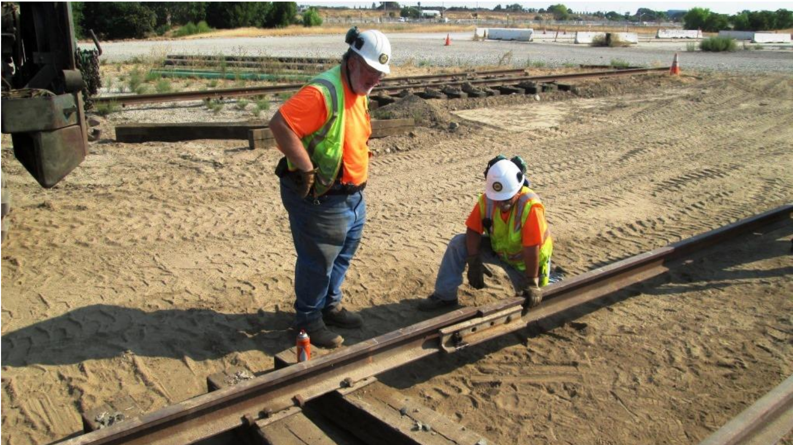
"Missed it by that much..." Frank and Joe contemplate the mismatch at the joint with the next panel of track...
