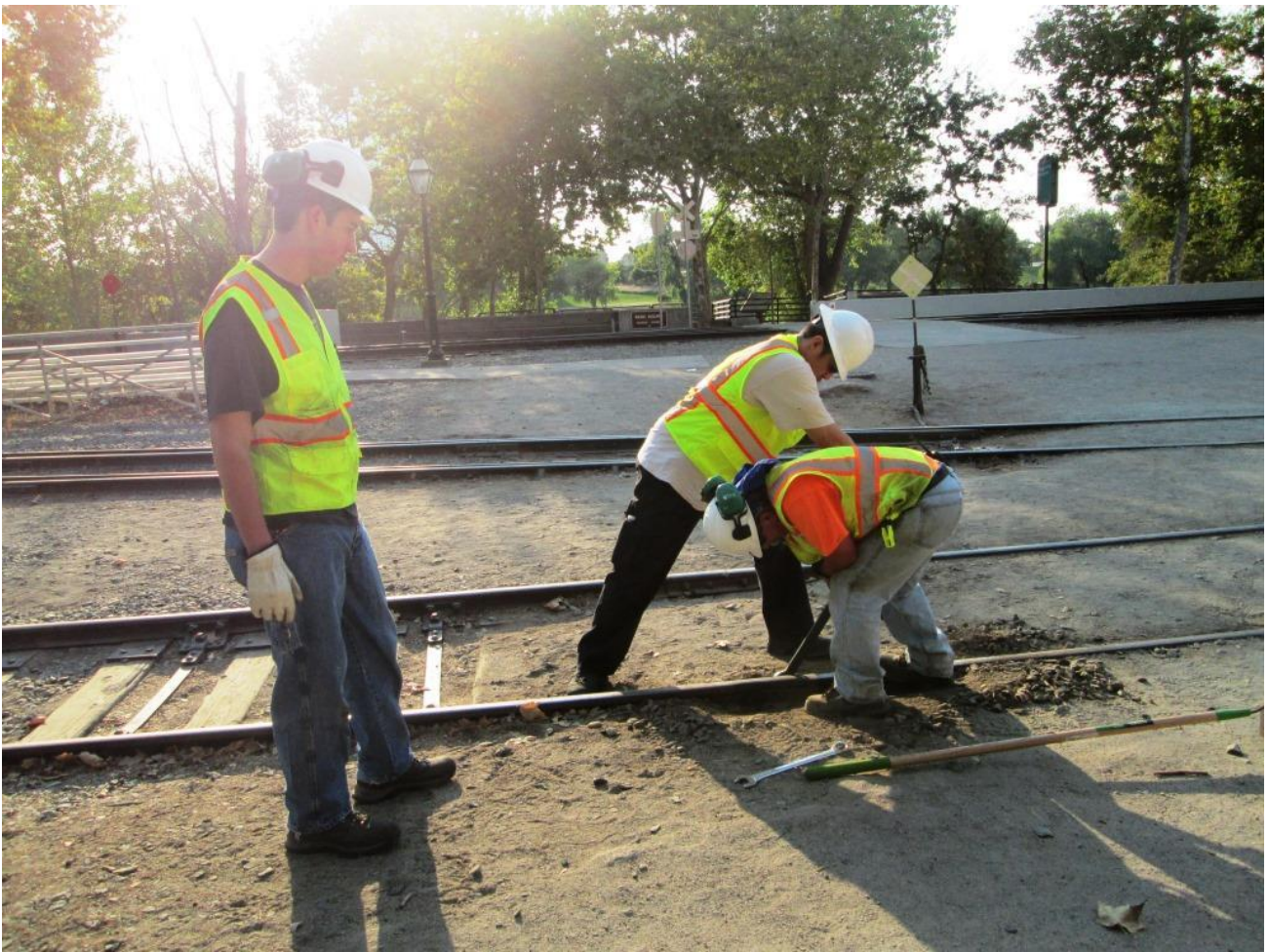
Weston, Jose, and Joe take on the jiggly-joint near the stub-switch
