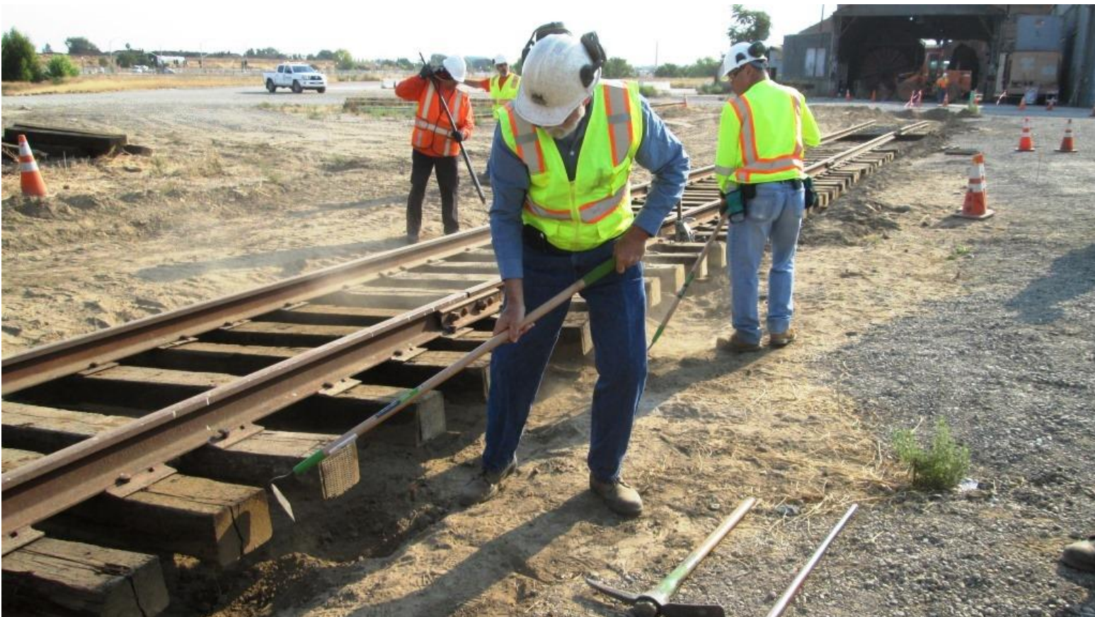
Alan and Taka use specially designed railroad dirt-moving tools
