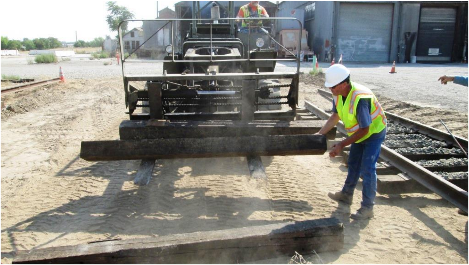
Andrew rolls ties off the forks of Big Green to position them for filling in the gap
