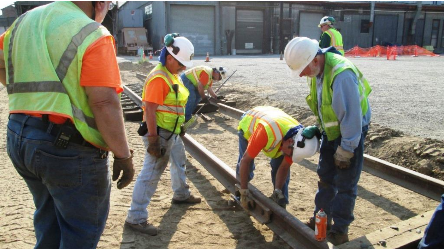
With the dancing done, everything is now in alignment. Joe, Ed, and Mike M. bolt the rails together
