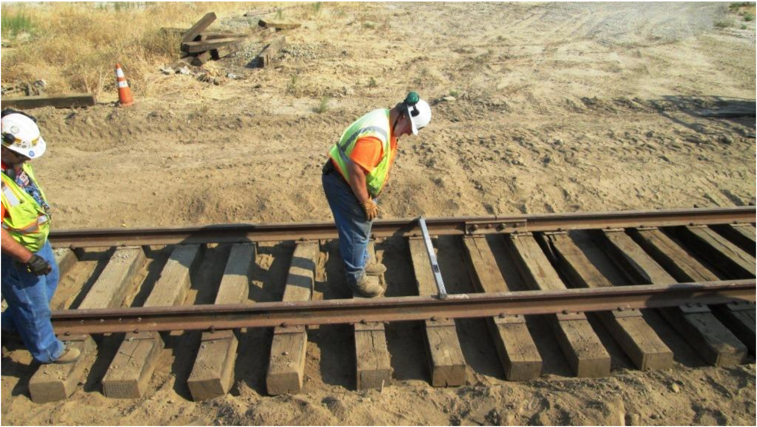
Frank checks the cross-level. "Spot on!" he declares
