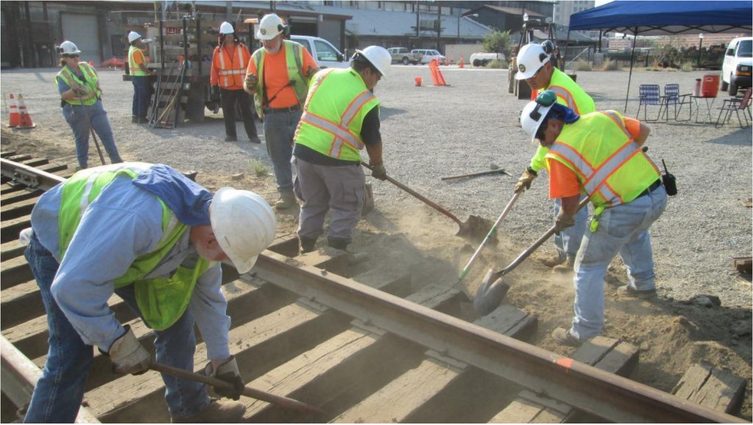
Dig ye tarriers, dig... Mike M., Anthony, Taka, and Joe are bound and determined to get this track level
