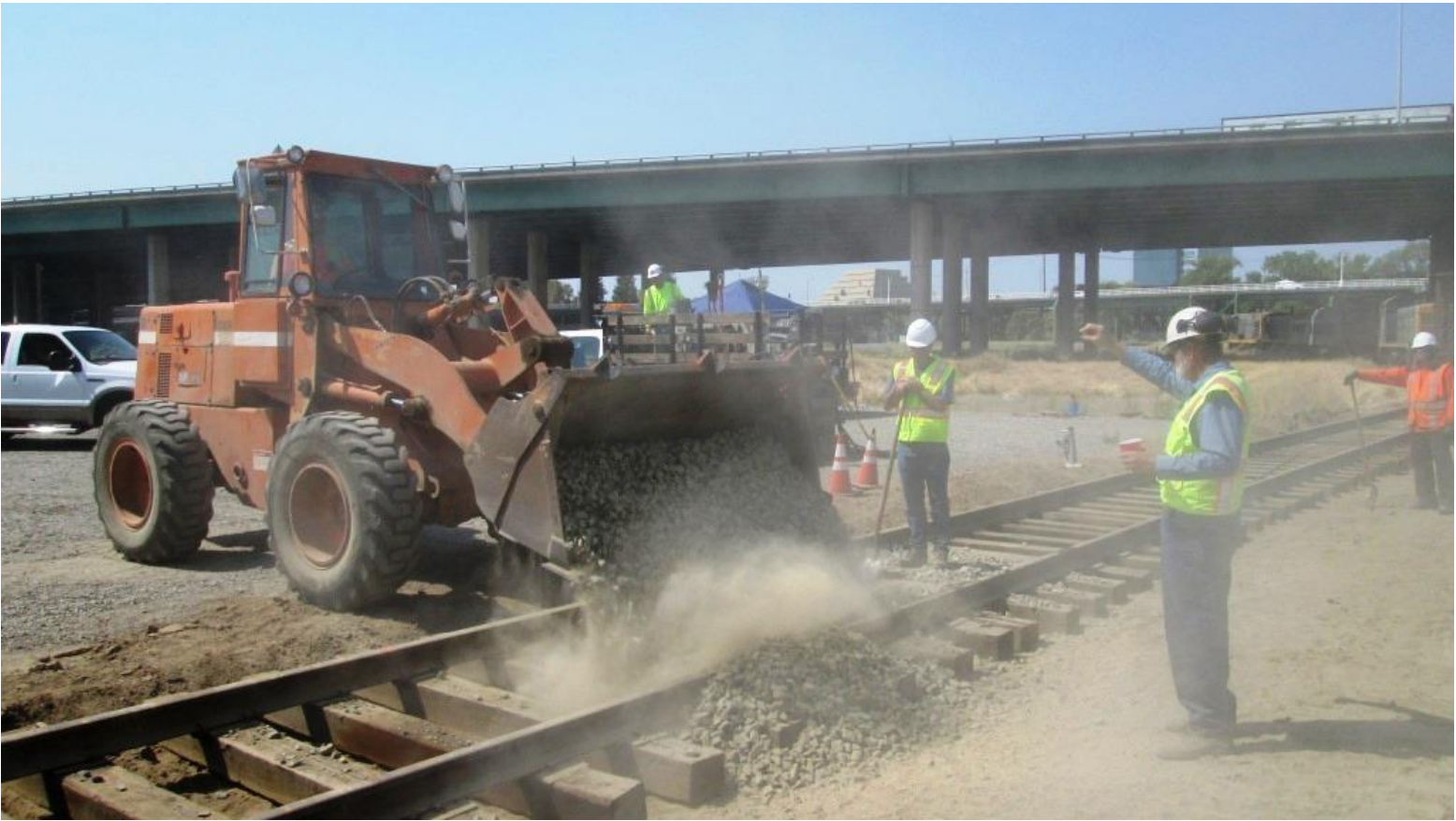
Frank bring in the first load of ballast rock
