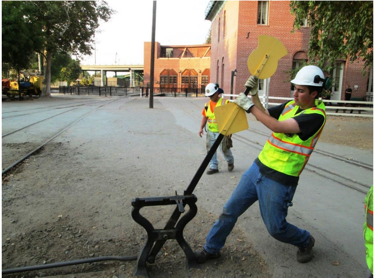
After servicing it, Weston tests the stub-switch
