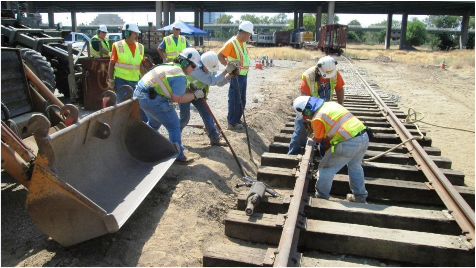
Team nipping: Heather and Mike M. nip-up the ties into which Mike F. and Joe are driving spikes
