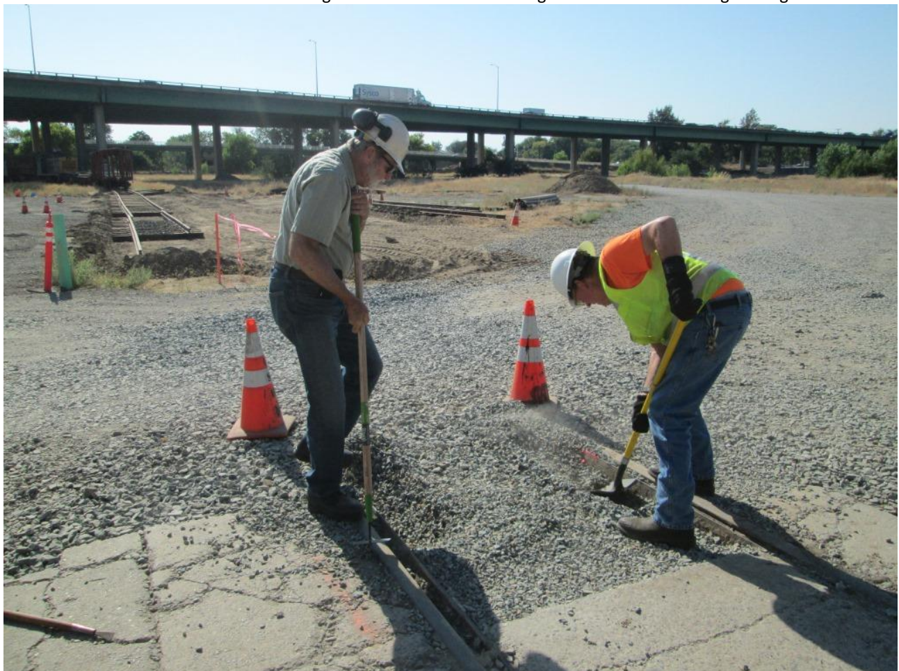
Alan and Cliff dig-out around the rails of the Firing Line Track to make room for cutting away the flange-guards
