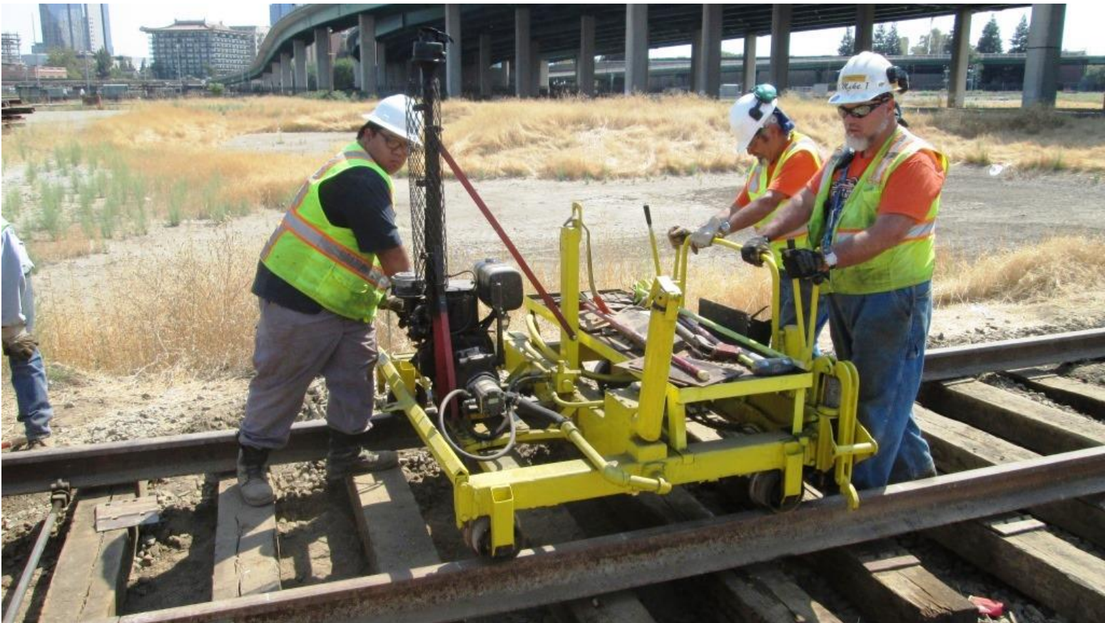
Anthony, Ed, and Mike F. deploy the rail-lifter for plating ties
