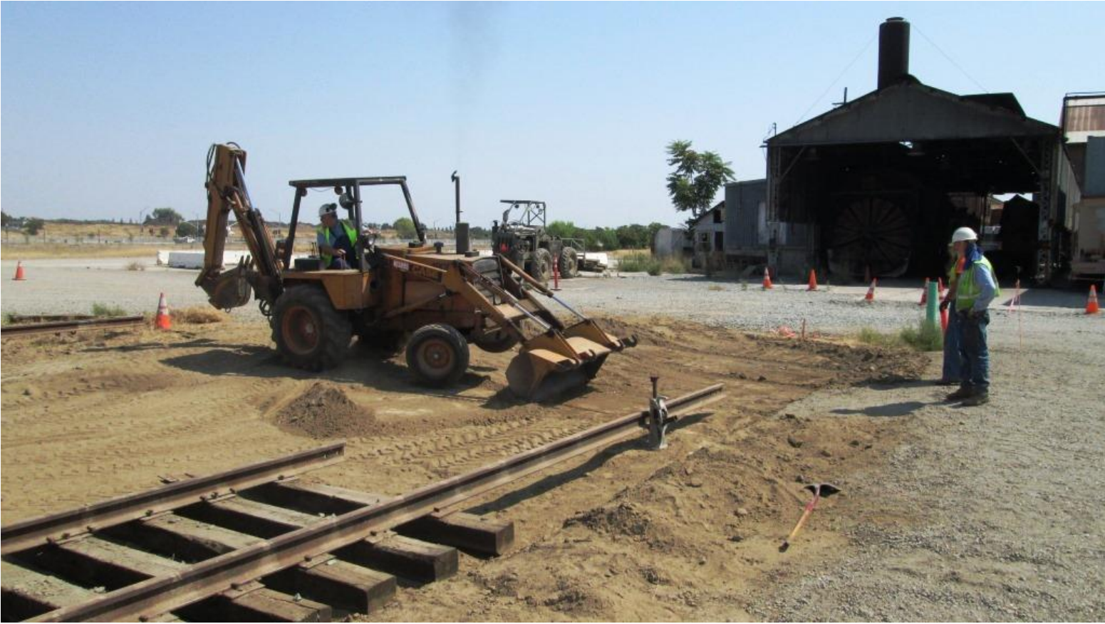
Chris uses the back-hoe as a grader
