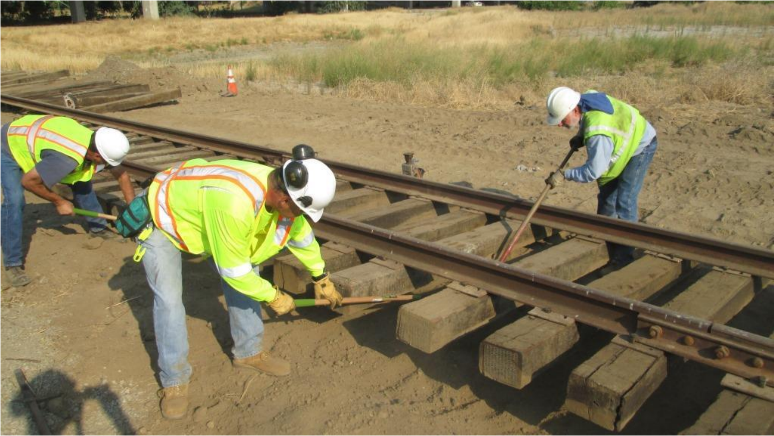
With the track levitating, Andrew, Taka, and Mike M. remove soil
