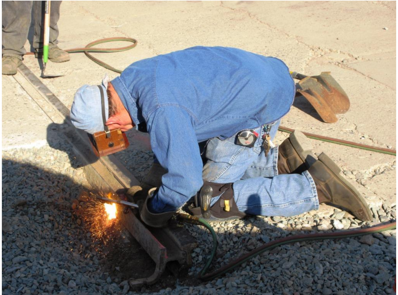
Cliff cuts the flange-guard off the rail to make room for drilling bolt-holes
