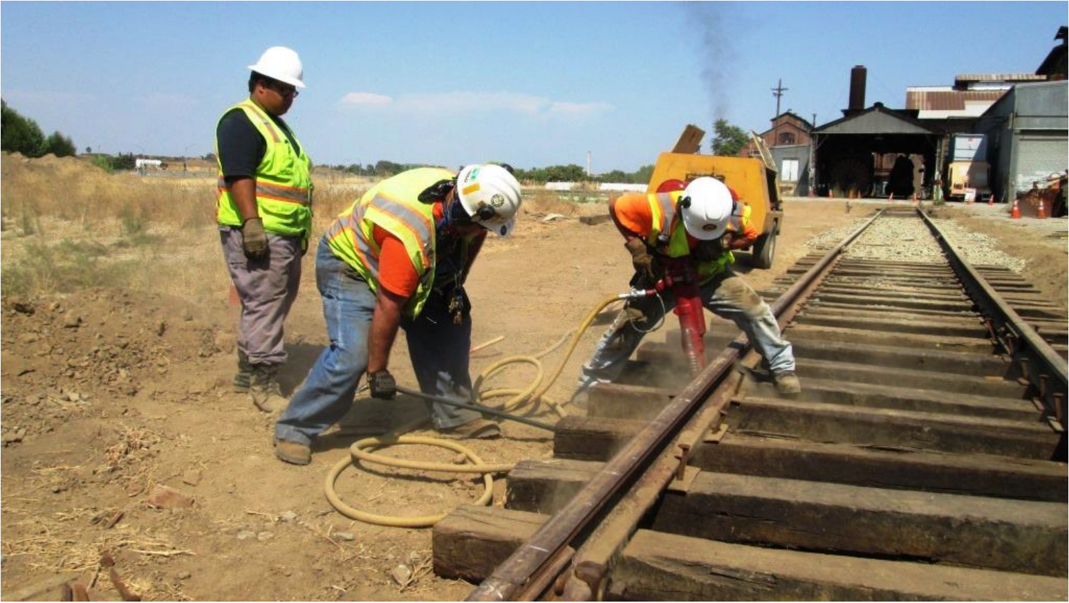
Mike F. nips-up the tie into which Joe is driving spikes
